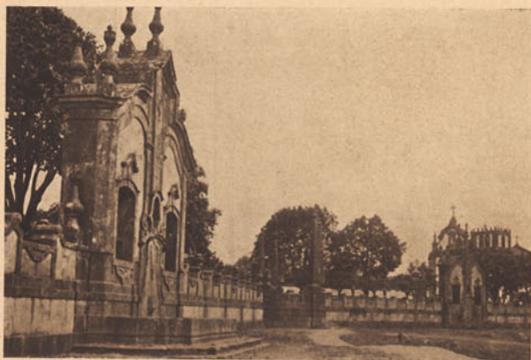
BARCELOS — AS OBRAS
